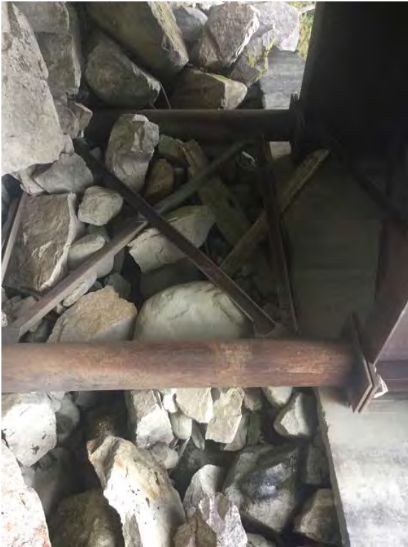
Left Bank Abutment when facing downstream
