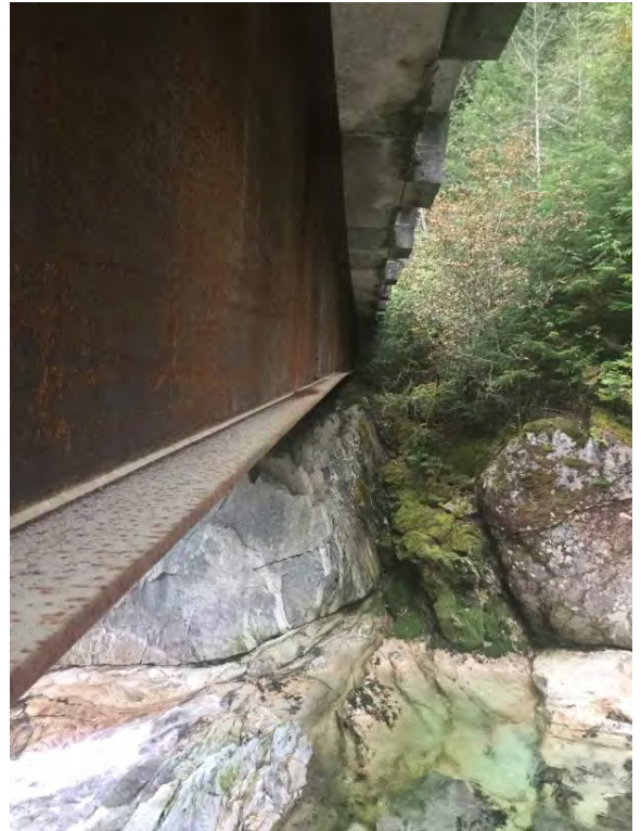
Upstream from Crossing
