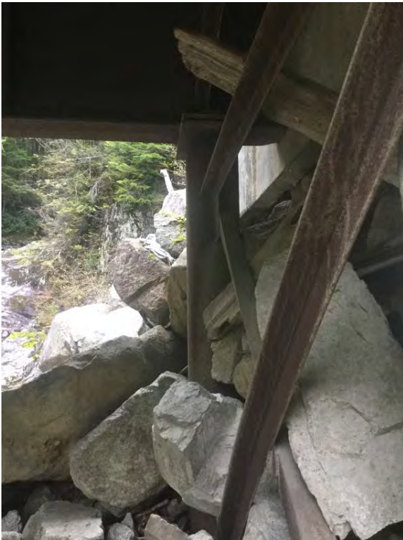
Left Bank Abutment when facing downstream
