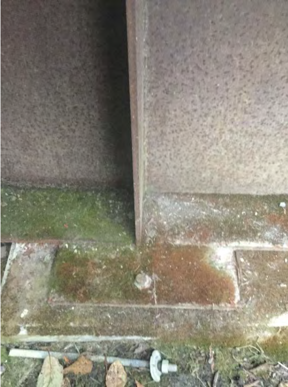
Right Bank Abutment when facing downstream
