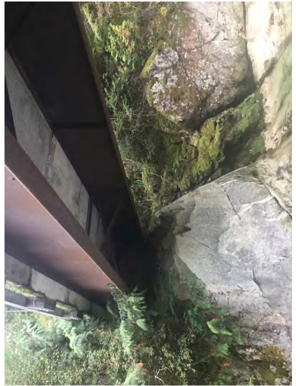
Right Bank Abutment when facing downstream
