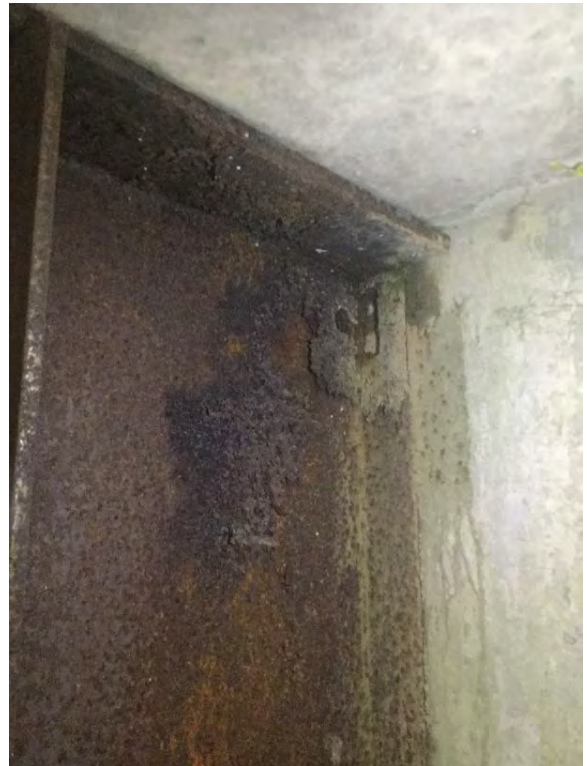
Right Bank Abutment when facing downstream
