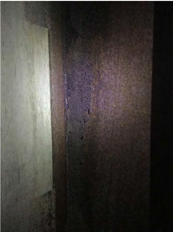
Right Bank Abutment when facing downstream
