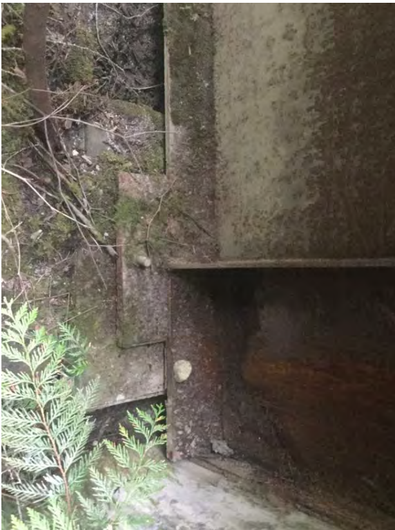
Right Bank Abutment when facing downstream - upstream side
