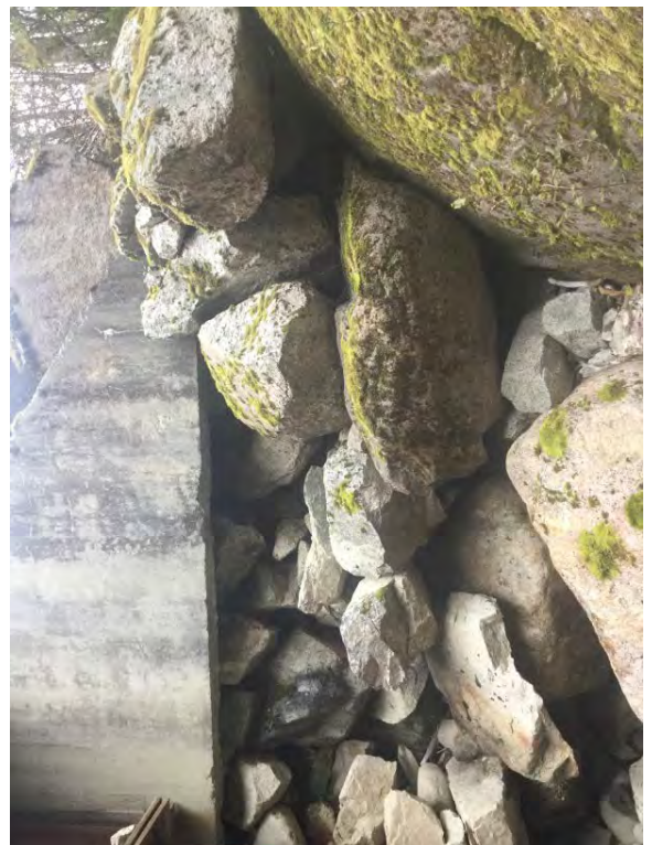
Left Bank Abutment when facing downstream
